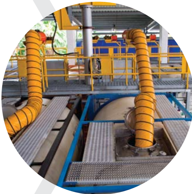
Having our very own fully automated, waste water treatment plant enables us to handle oil base and chemical cargos.
